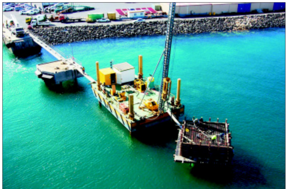
All tied up: Work is already well advanced on construction of a new mooring dolphin at Burnie terminal to accommodate the longer vessels. (Photo: Courtesy Captain Mark Dudding)
